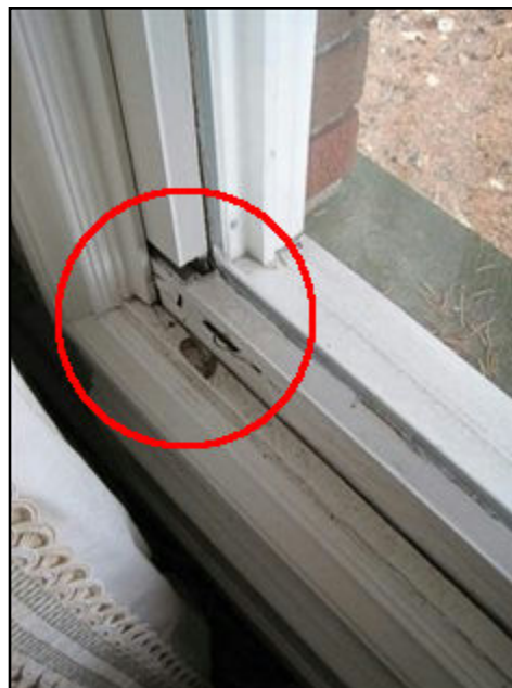
27. Significant rot at living room window.
