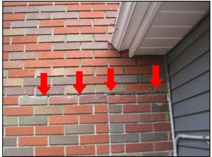
12. Re-point brick joint in back (fill w/mortar)
