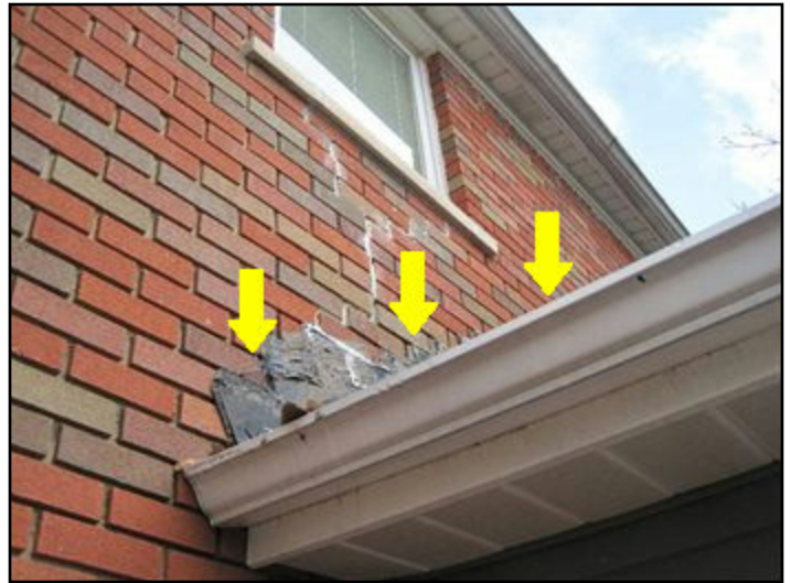
4. Re-flashing or re-tar flashing at addition.
